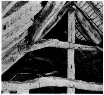
FIG. 1. The upper part of the closed truss over the Hall.
