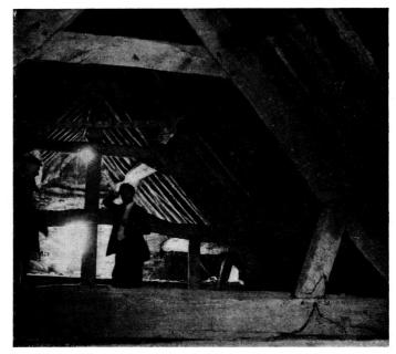
FIG. 2. Open truss in the foreground, showing massive baulk-tie.
